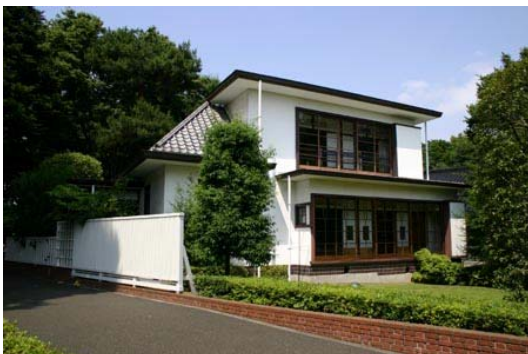
Japanese "Prairie Style" house, 1925 Edo-Tokyo Open Air Architectural Museum
